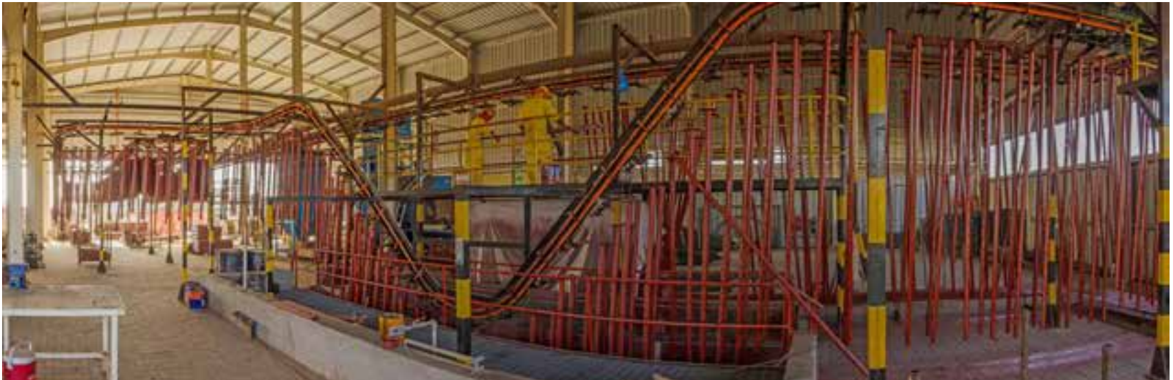
Maintenance & refurbishment with automated painting line
