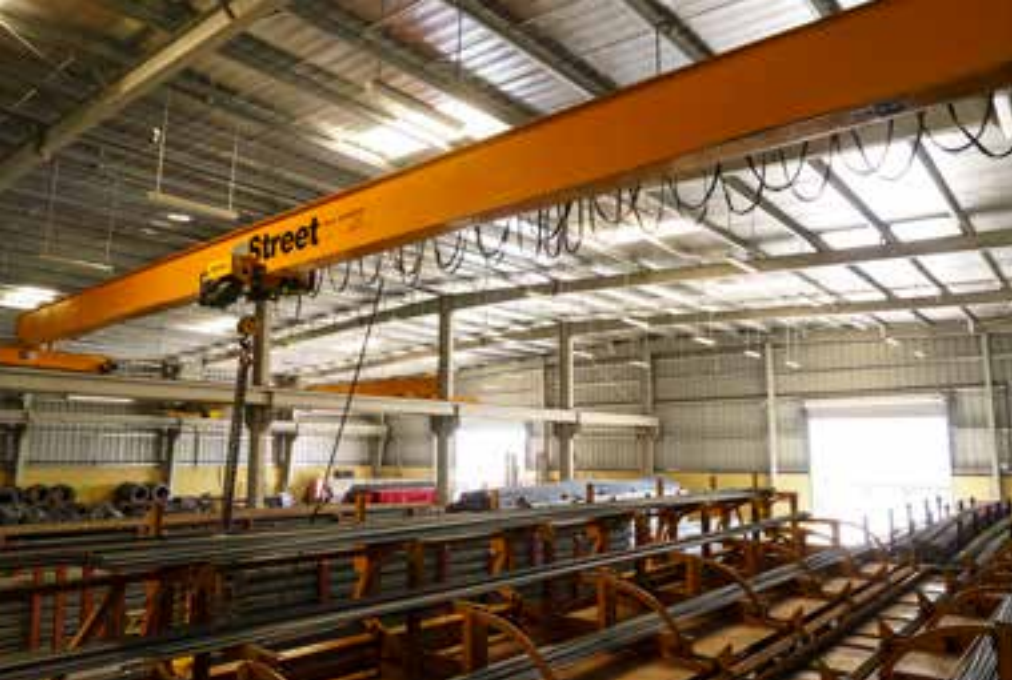
Steel Fabrication unit
