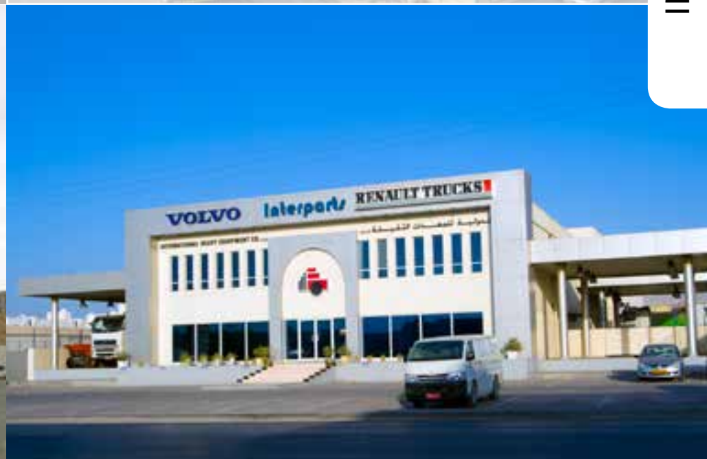
Showroom and service center for Volvo at Muscat
