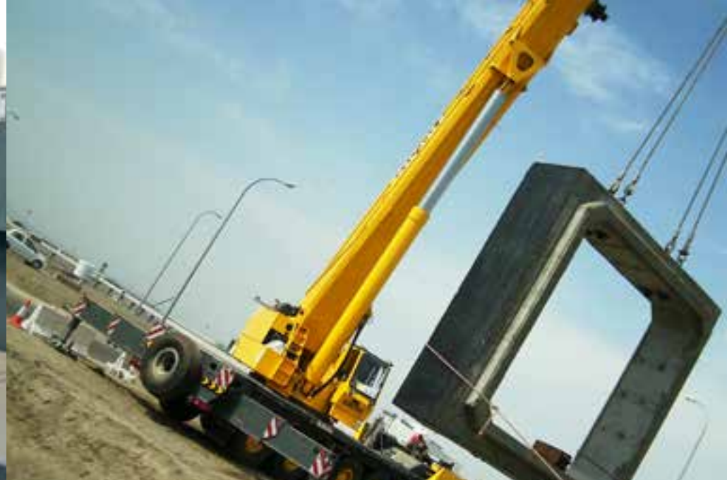
Culvert size 3X3 mtrs for road crossing
