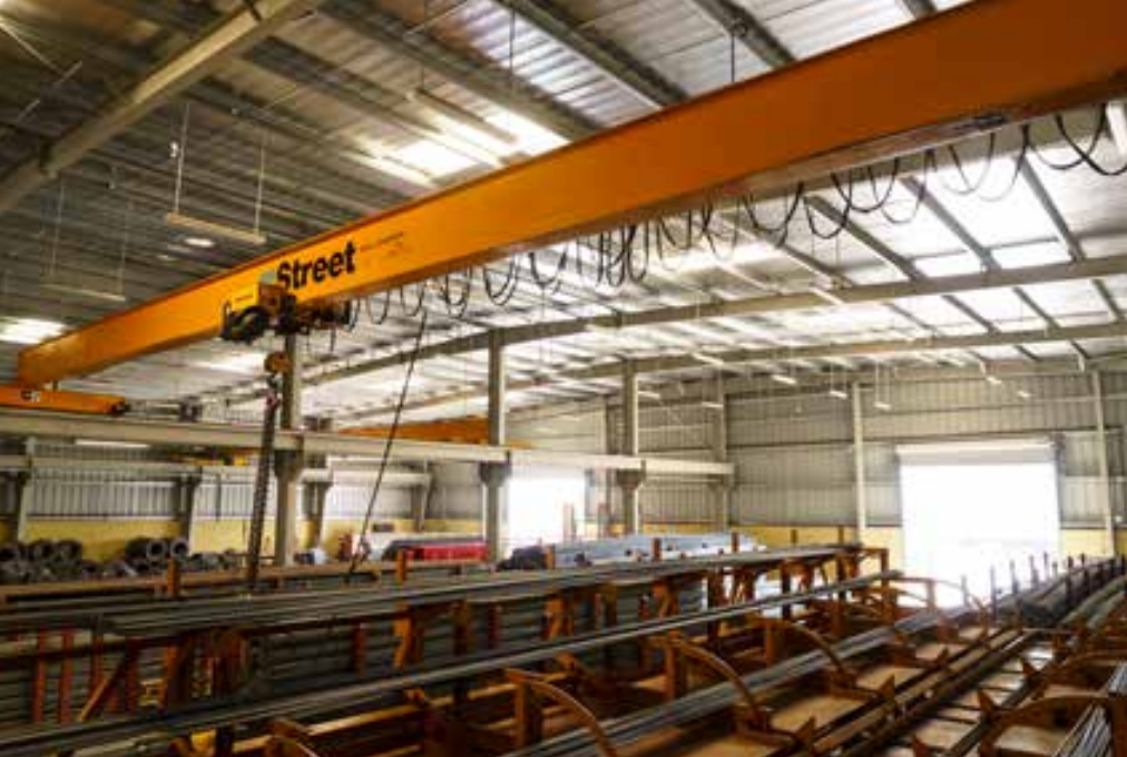
Steel Fabrication unit
