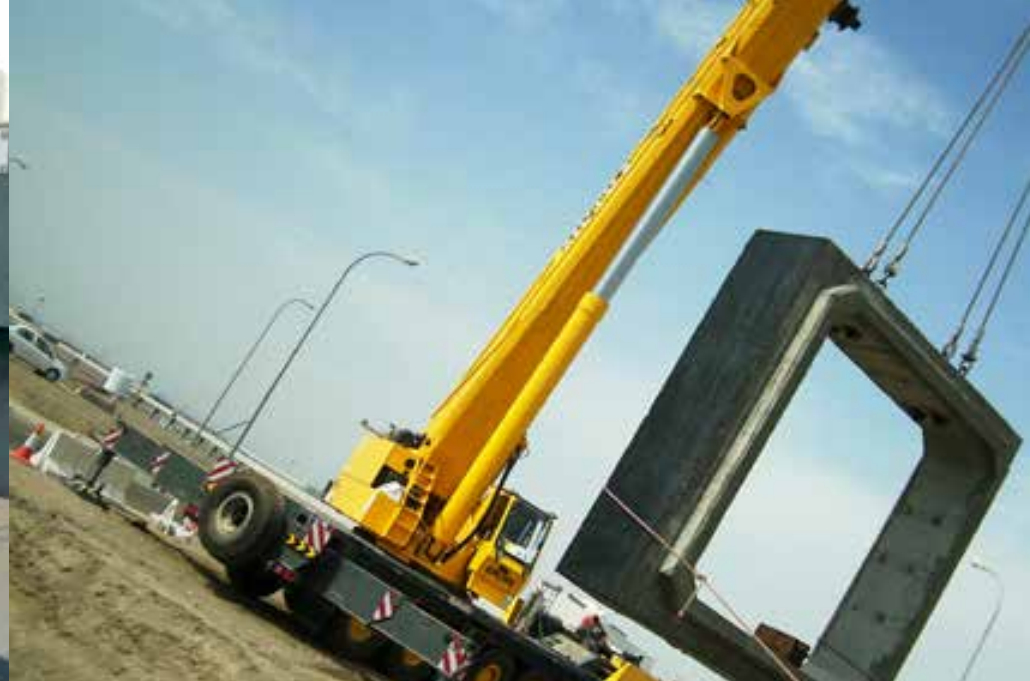
Culvert size 3X3 mtrs for road crossing
