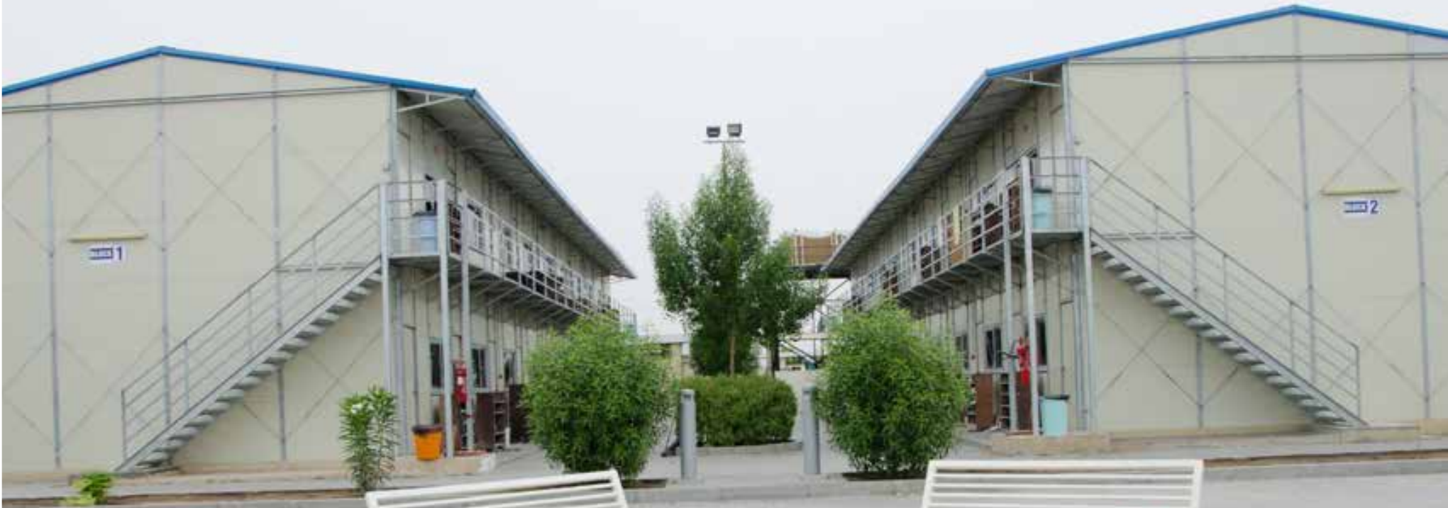
Workers accommodation complex
