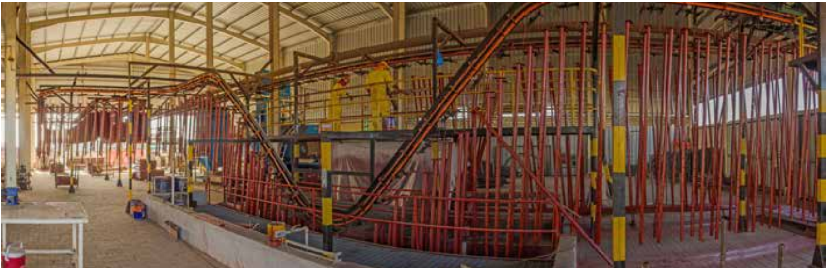
Maintenance & refurbishment with automated painting line
