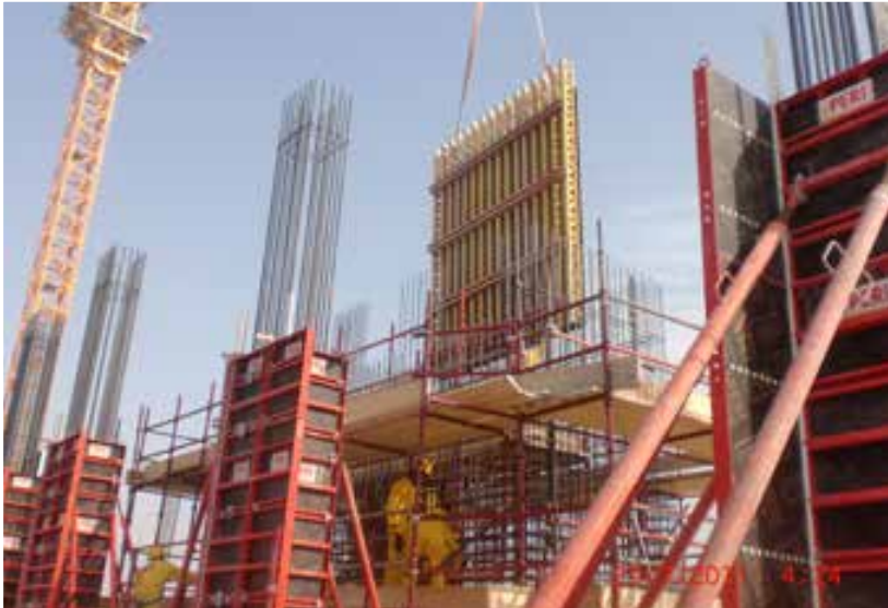
Proprietary solutions from DOKA & PERI
